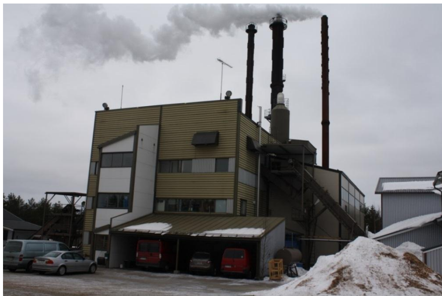
Figure 10. Siikaranta district heating plant in Suomussalmi.
