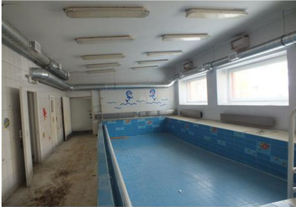
Figure 20. The entire swimming pool, after repair.
