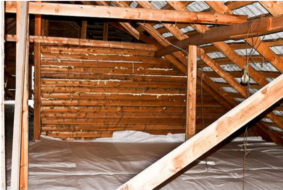
Figure 25. Attic of the kindergarten after repair. Isolations of the ceiling, walls and floor are shown in photo.
